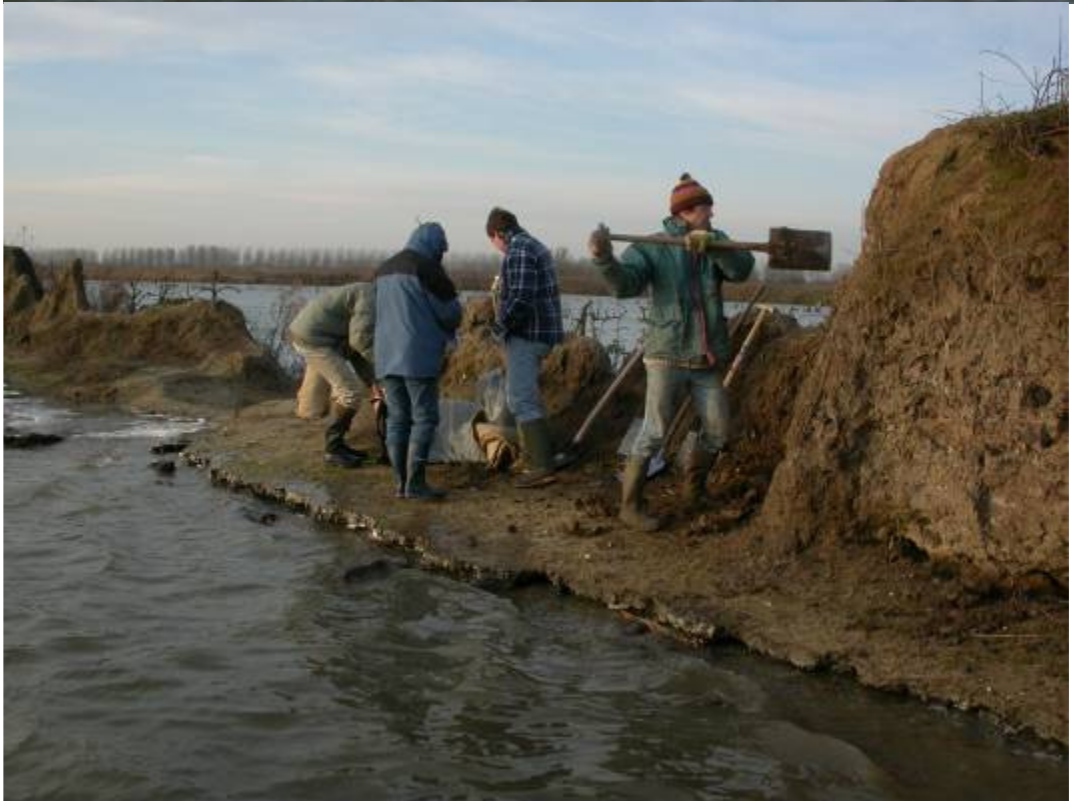
Figure 7 & 8: Volunteers creating an artificial nest site and repairing a dike (Verrebroek, 15/03/2009).
